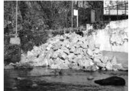
The City acted quickly to repair damage to Falls Road.
