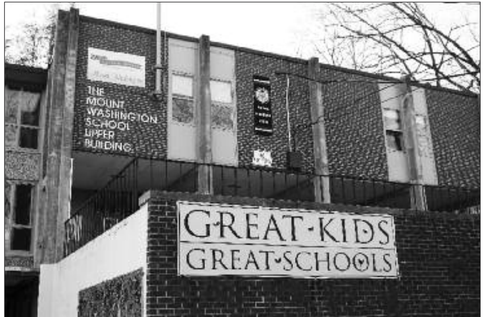
The Mount Washington School building would receive extensive renovations under the City Schools plan.
